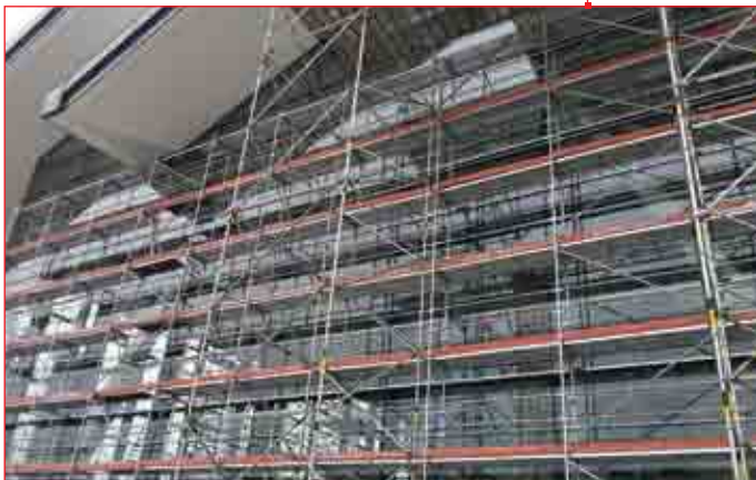
Works at the airport building facade
