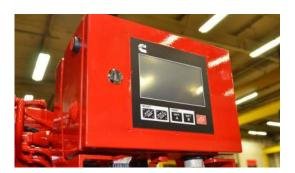
The Cummins FPDP is an integrated microprocessor-based control system that provides full digital technology with enhanced accuracy and built-in redundancy.
