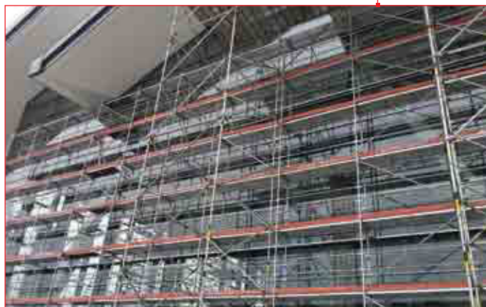
Works at the airport building facade
